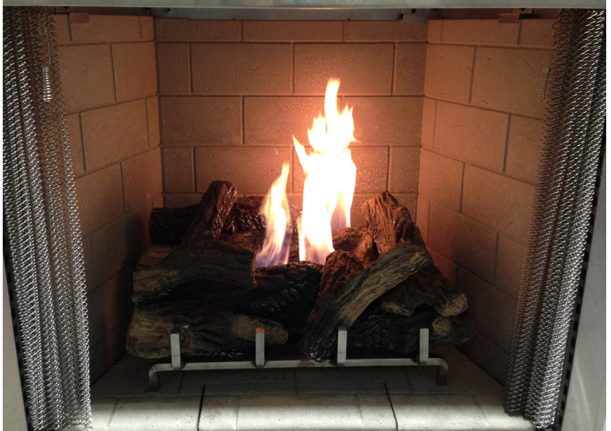
Figure 23 - Proper Burner Flame Appearance
