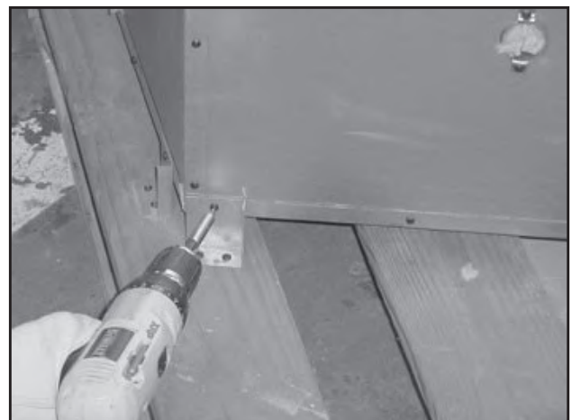
Figure 3.12 Removing Shipping Brackets
