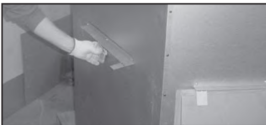
Figure 3.7 Bending Refractory Shipping Tabs Back Down
