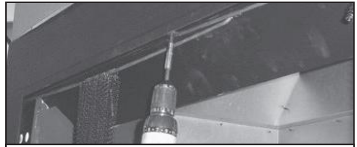
Figure 3.9 Removing the Screen Rods
