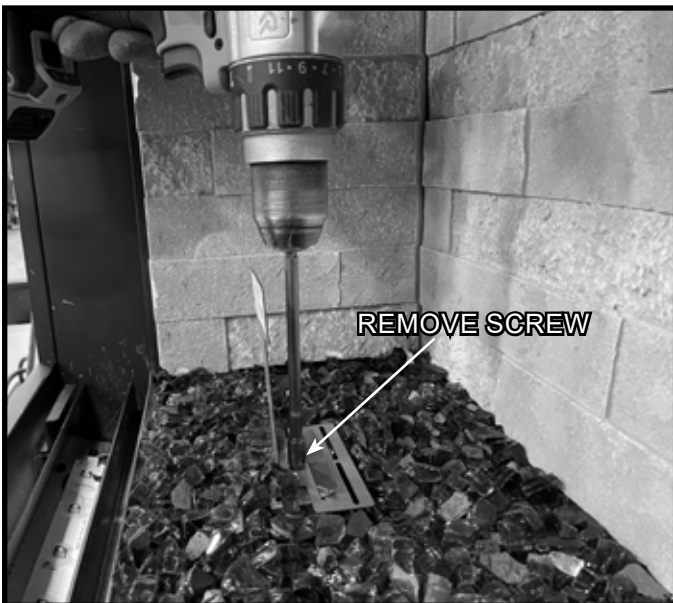
Figure 11.4 Place Media, Remove Media Placement Jig Screw
