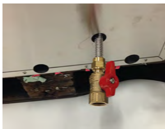
Figure 12 Gas connection
