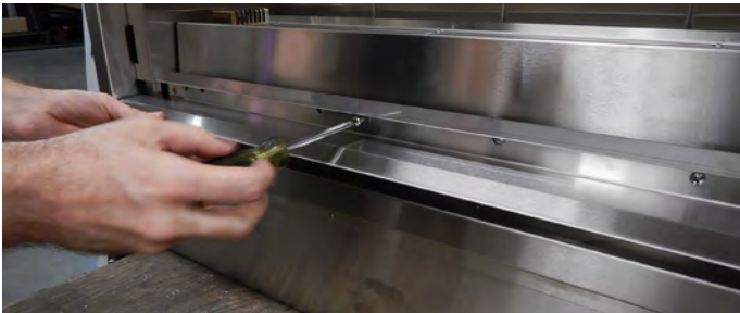
Figure 4 Removal of lower air baffle
