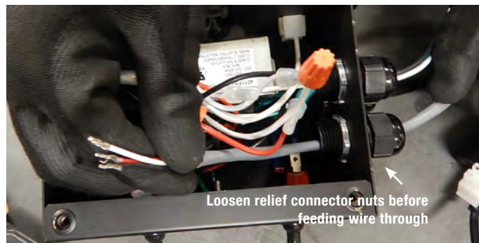
Figure 37 Feeding the wire through the control box
