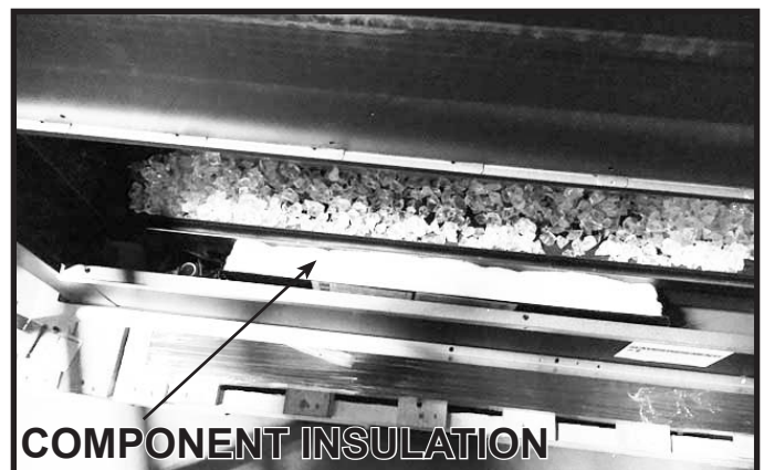
Figure 11.3 Component Insulation Location
