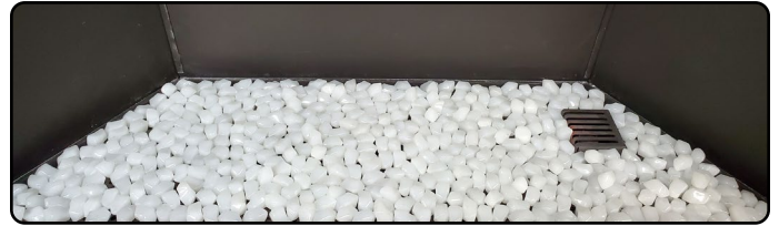
Figure 24.bb Completed firestone installation
