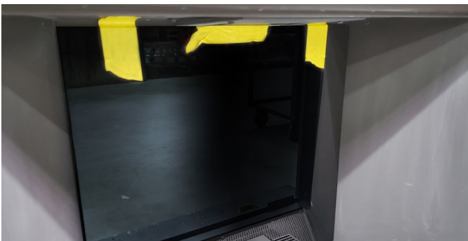
Figure 20.b hold it in place using masking tape
