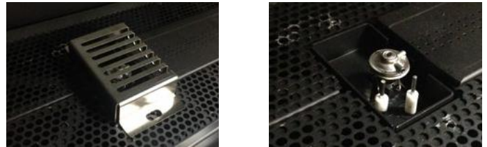
Figure 13. Removal of pilot cover
