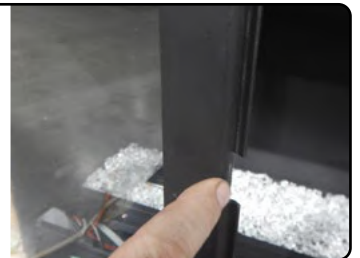
Figure 21.b Installing the door
