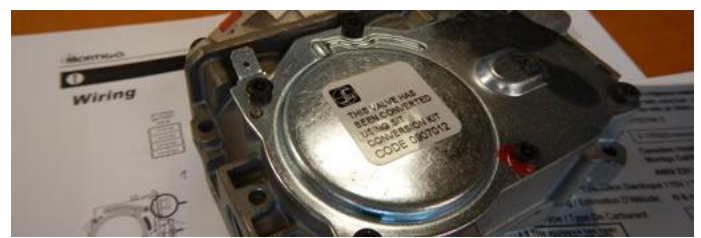
Figure 13.k Conversion label on valve
