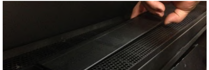
Figure 13.b Loosening the venturi
