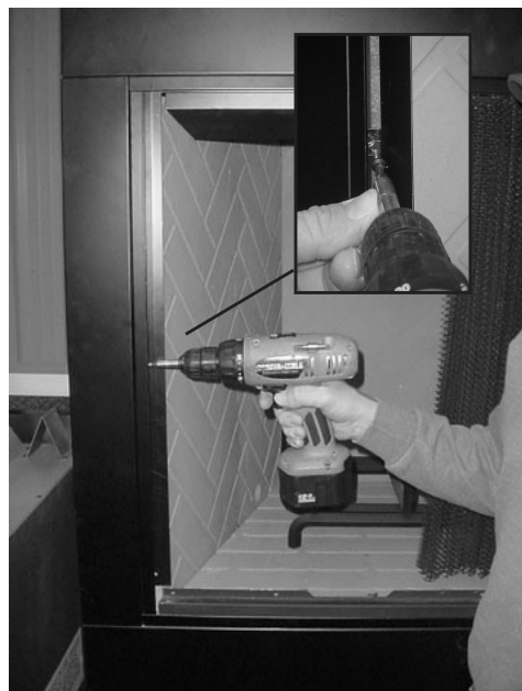
Figure 5 - Fastening the Side Filler
