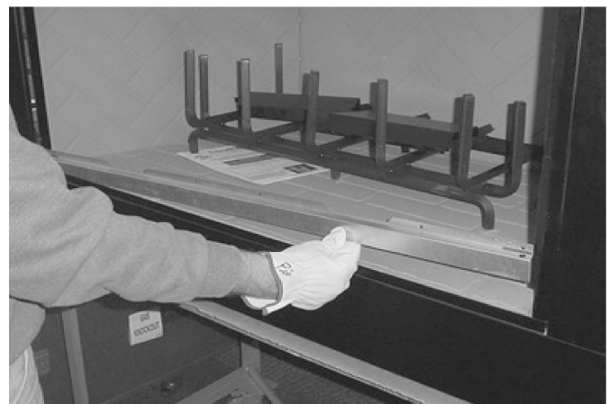
Figure 1 - Install the Door Track
