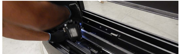
Figure 13. Removal of burner strip
