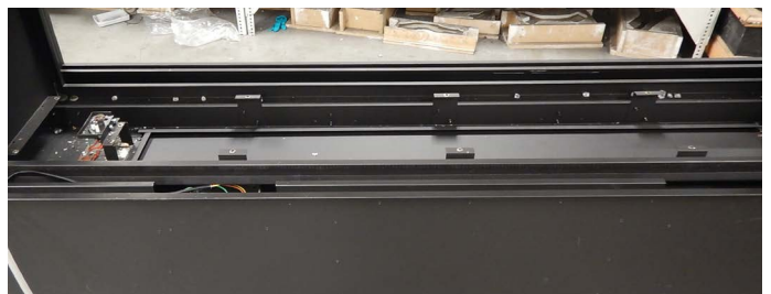
Figure 12.e Removing the Burner
