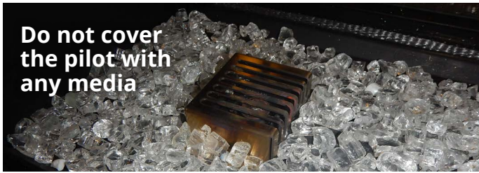
Figure 22. Do not cover the pilot with any media
