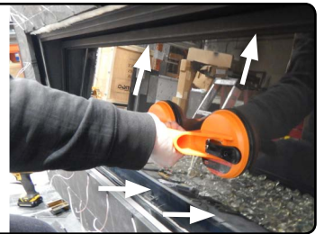
Figure 21.b Installing the door
