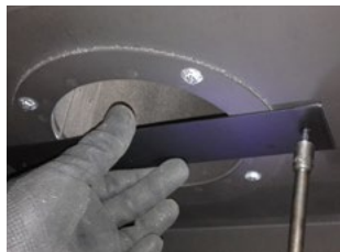
Figure 8.b.c Restrictor plate Installation
