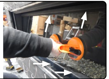
Figure 21.b Installing the door
