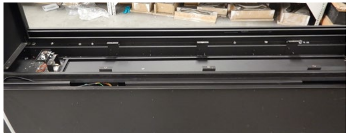
Figure 12.e Removing the Burner
